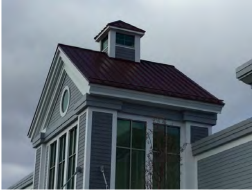
STANDING SEAM ROOF
