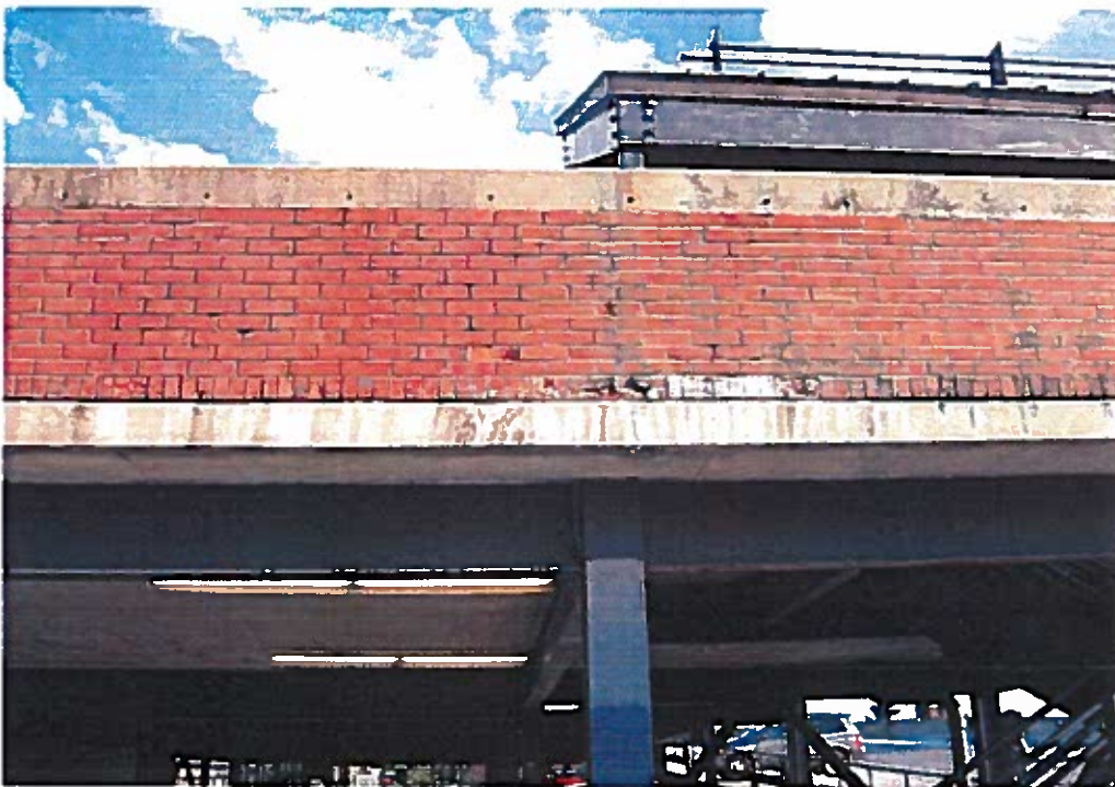
Deteriorating brick @ 5 th level, north side.
