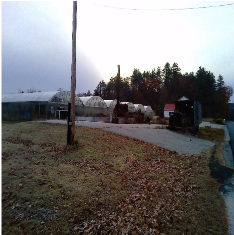
115 River Road West face of Greenhouses
