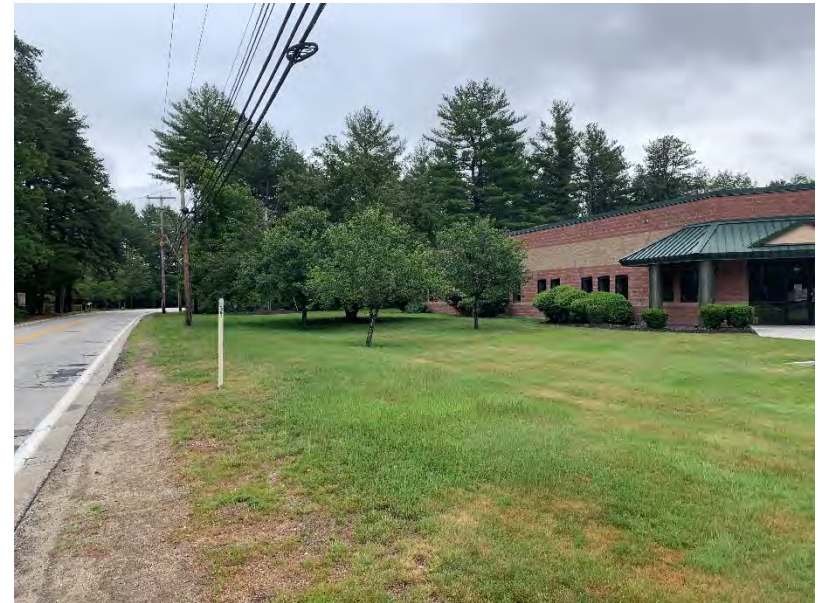
Figure 8: (2021-06-15) Southeastern view of the existing building front where proposed sidewalk shall be constructed around the building.
