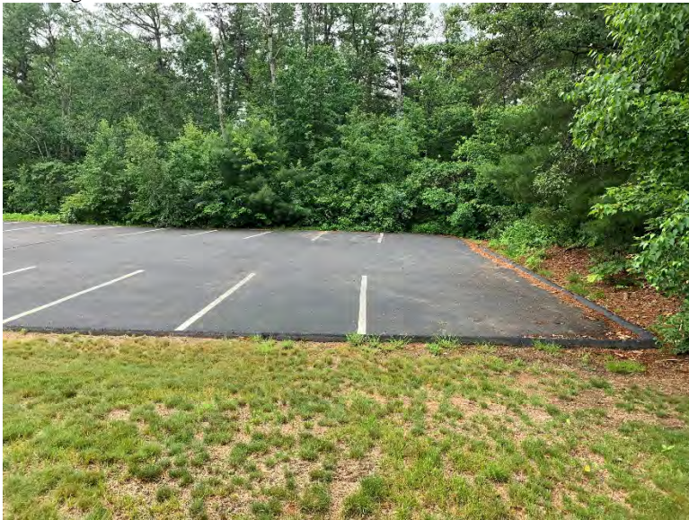
Figure 3: (2021-06-15) Extent of existing pavement of western parking lot.
