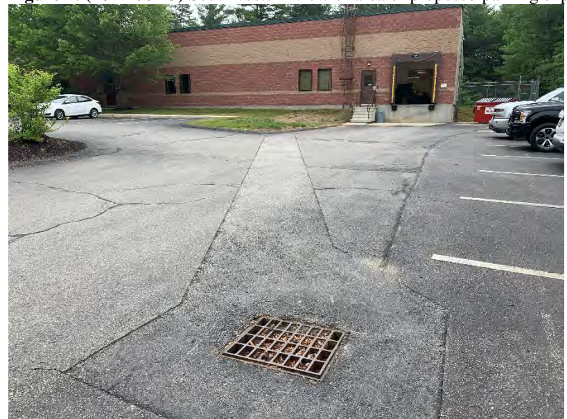
Figure 4: (2021-06-15) Eastern view of southern side of building with existing catch basin.
