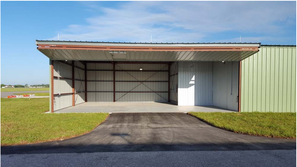
Picture 2: Front View of Hangar Interior
