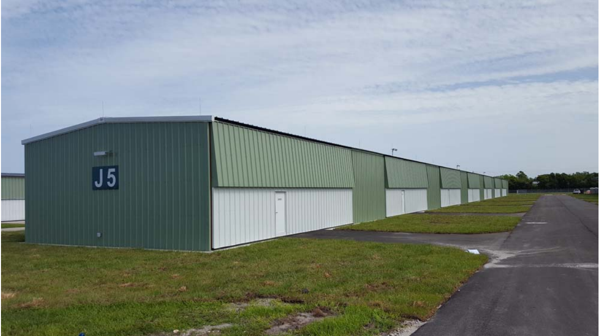
Picture 1: Exterior of Hangar
