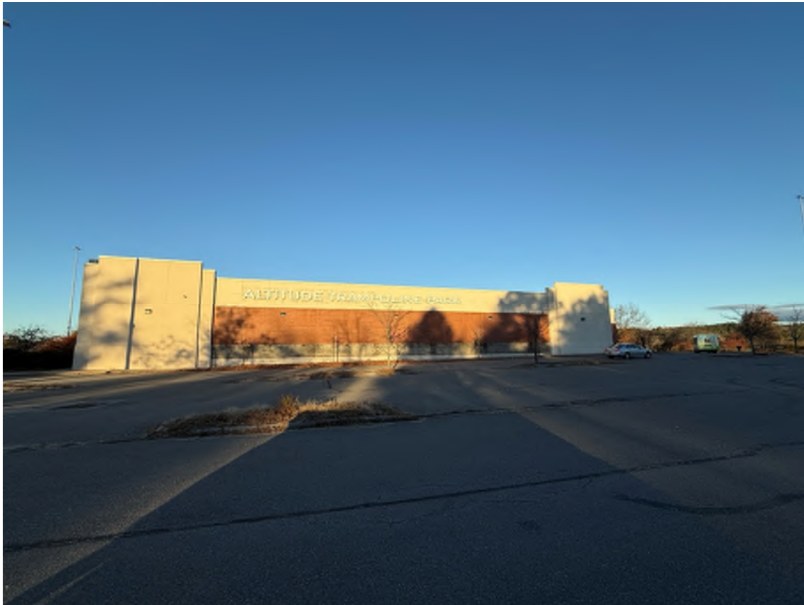
Photo 17: Looking West at the East end of the mall (building to remain).
