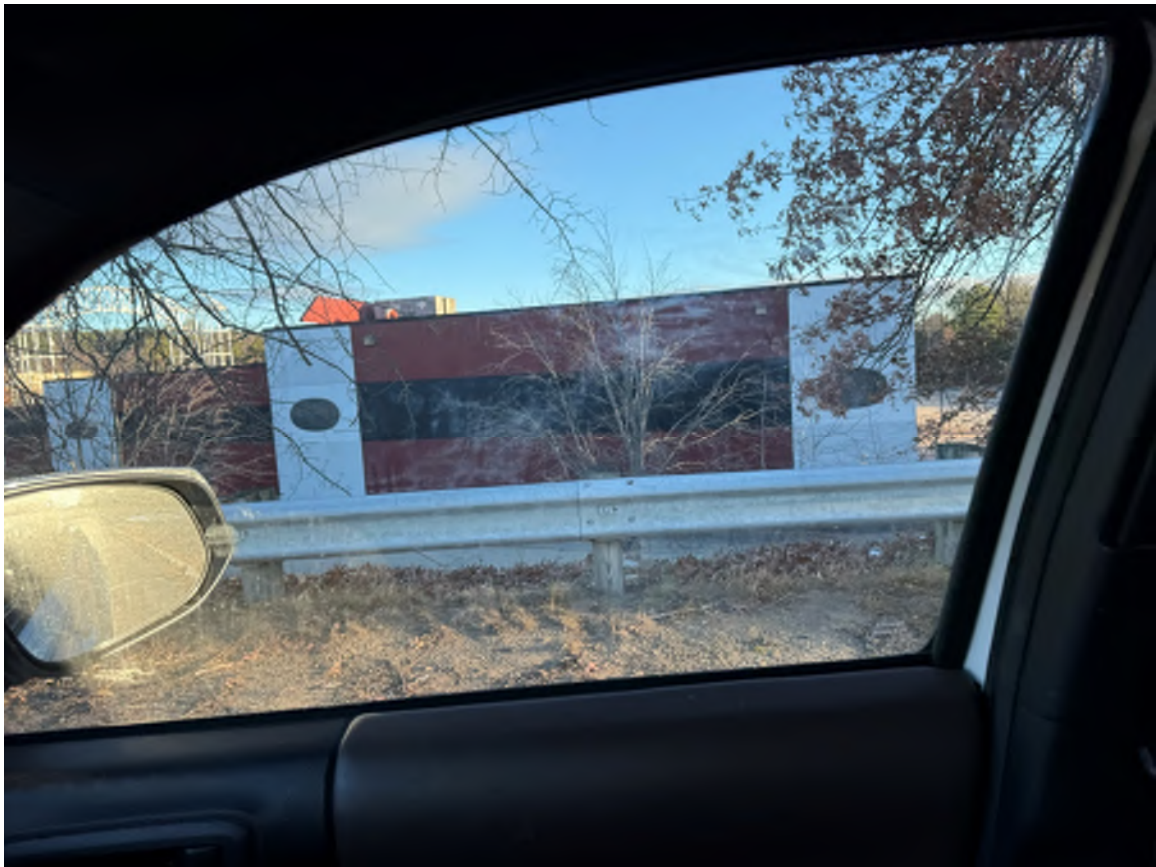
Photo 20: Looking North at the South side of Cinema (building to be razed).
