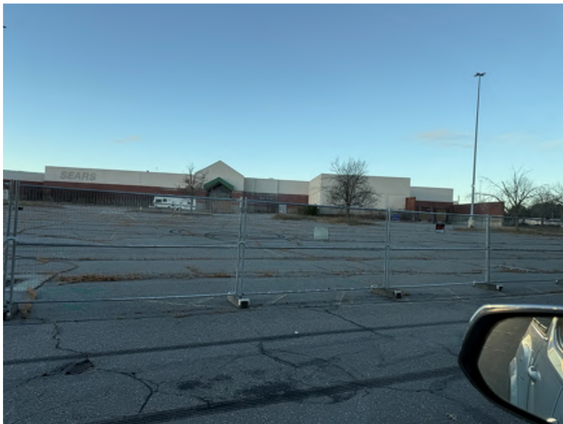
Photo 6: Looking South at the North-East corner of the mall (building to be razed).
