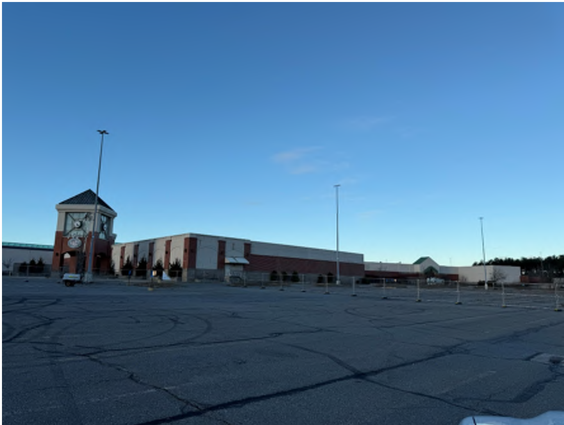
Photo 5: Looking Southwest at the North-West side of the mall (building to be razed).
