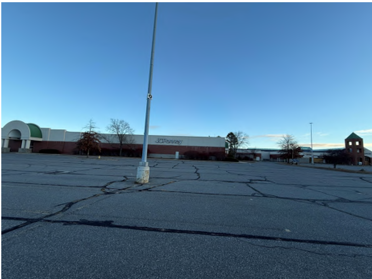
Photo 14: Looking North at the South side of JC Penney (building to be razed).
