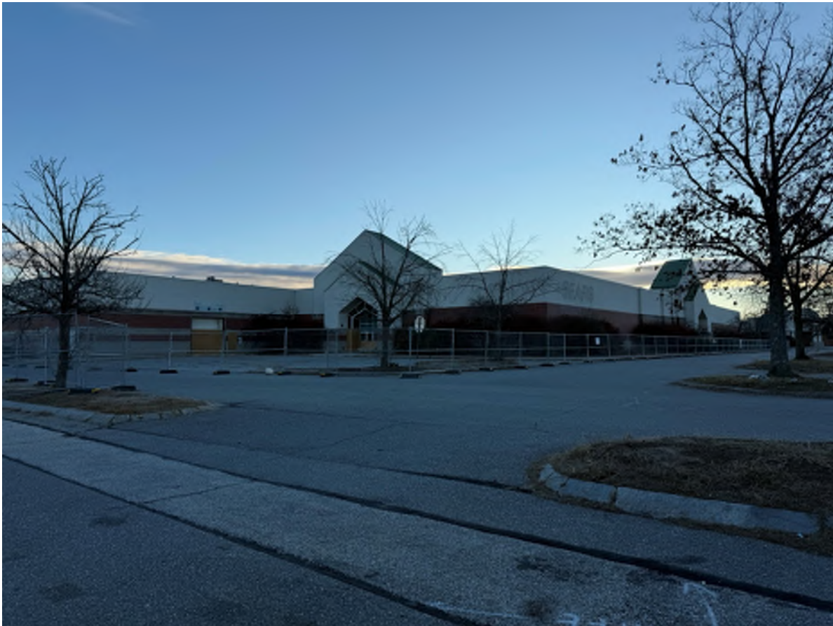
Photo 9: Looking Northeast at the South-West corner of the mall (building to be razed).
