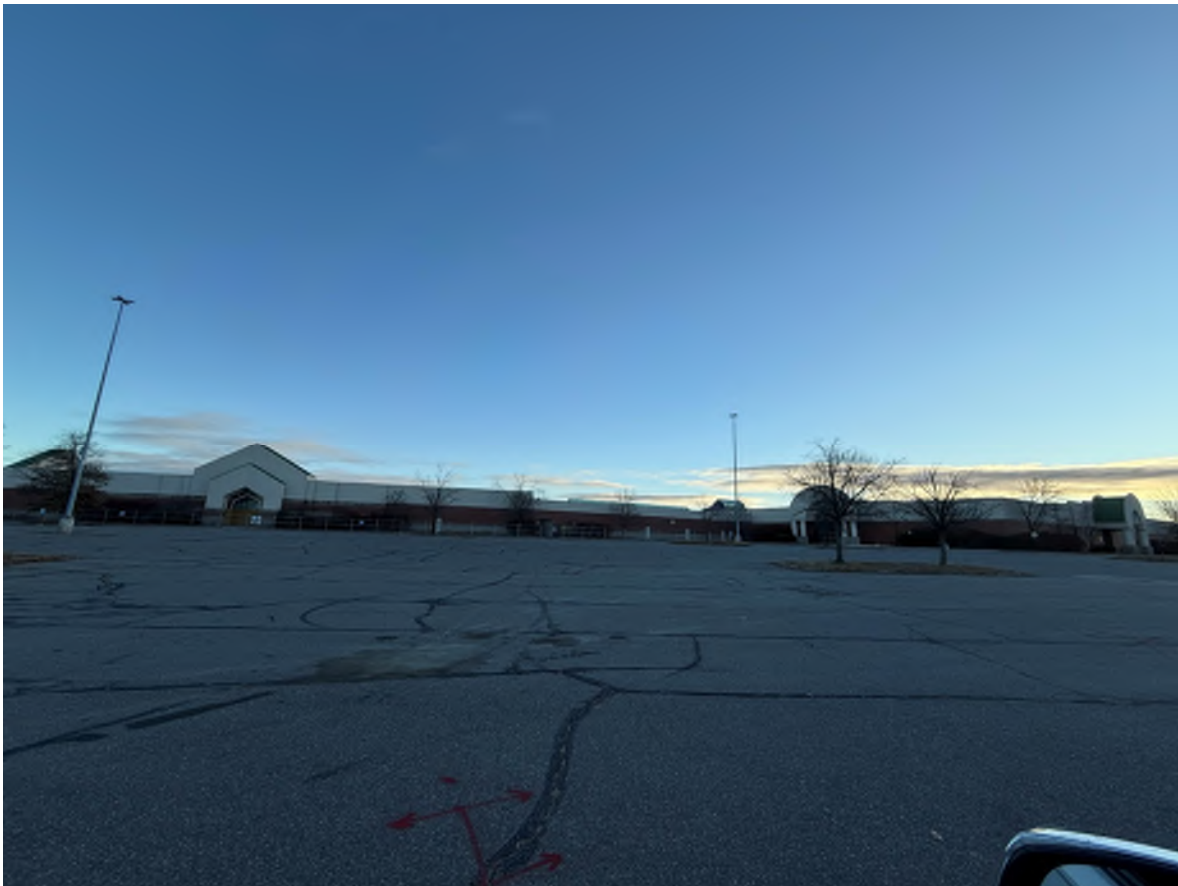
Photo 13: Looking North at the West end of the mall (building to be razed).
