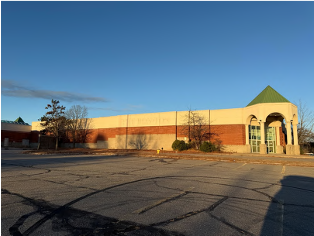
Photo 2: Looking Southwest at the Northern Portion of the mall (building to be razed).
