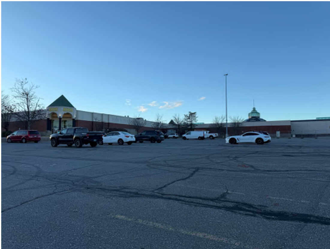
Photo 4: Looking Southeast at the Northern-Middle portion of the mall (building to be razed).
