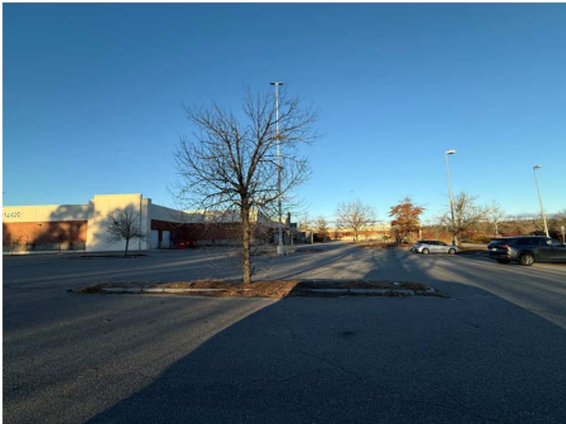
Photo 18: Looking West at the Northeast corner of the mall (building to remain).
