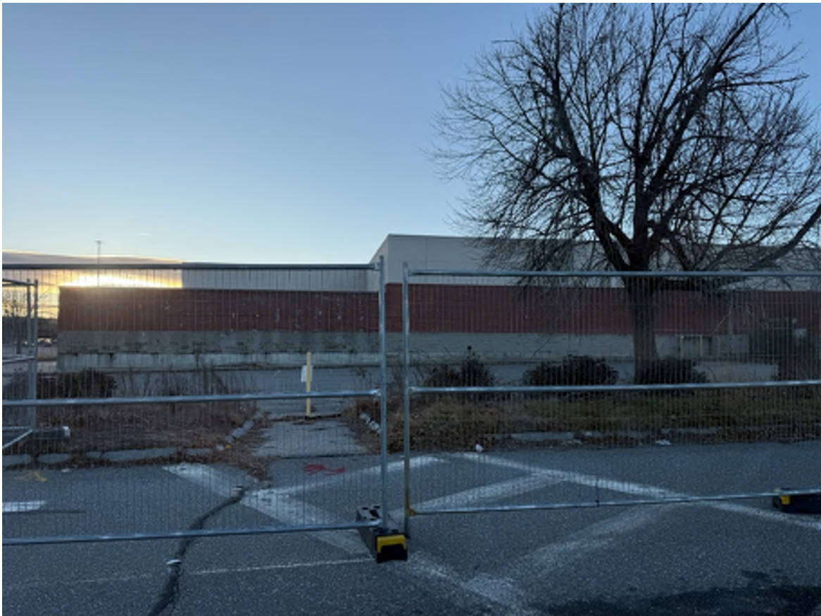
Photo 7: Looking East at the North-East corner of the mall (building to be razed).
