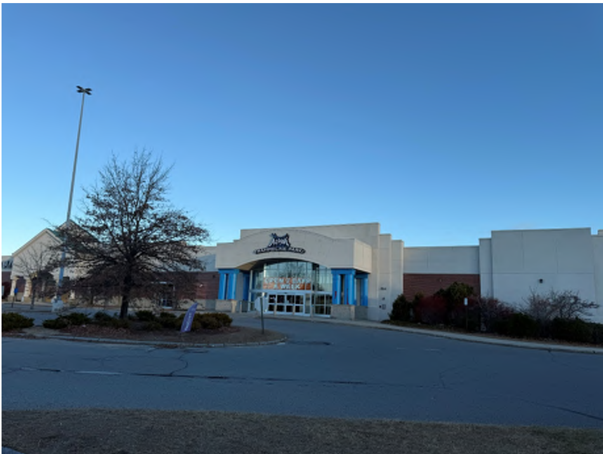
Photo 16: Looking Northwest at the Southeast corner of the mall (building to remain).
