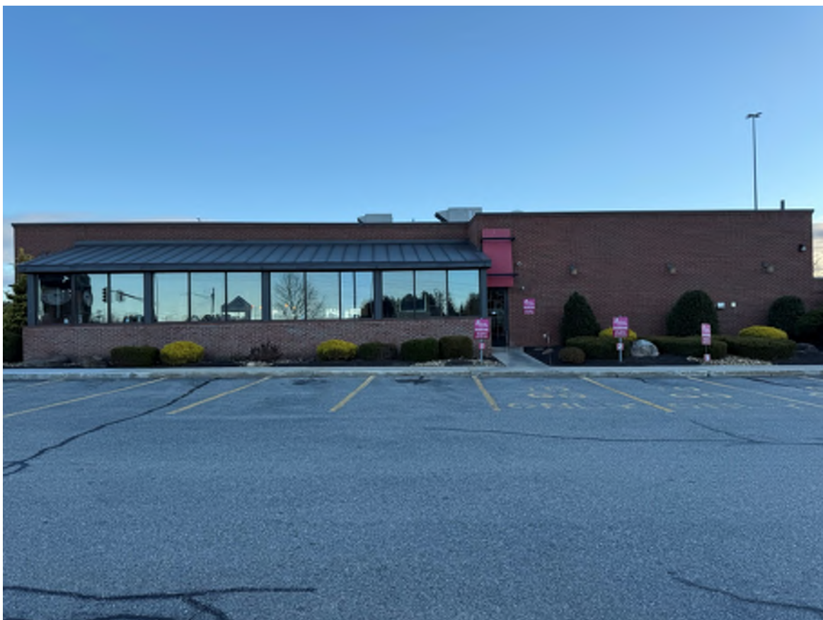
Photo 12: Looking North at the South side of Applebee's (building to remain).
