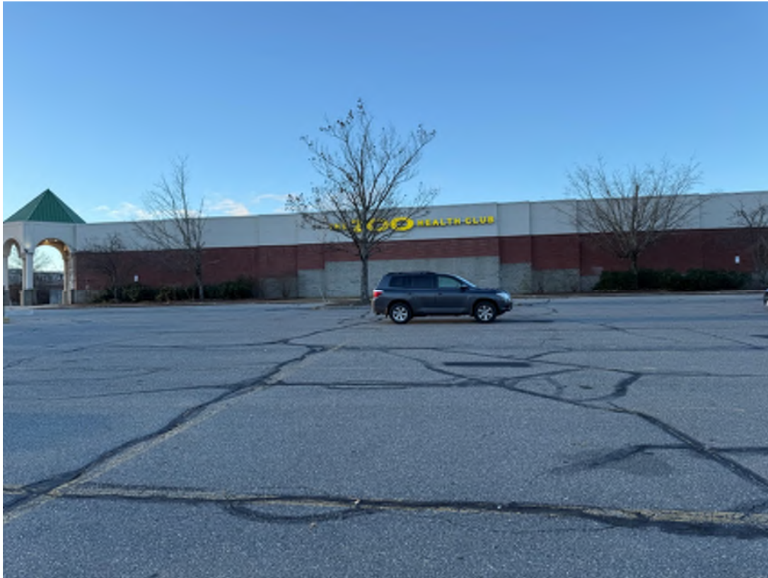
Photo 3: Looking South at the Northern-Middle portion of the mall (building to be razed).
