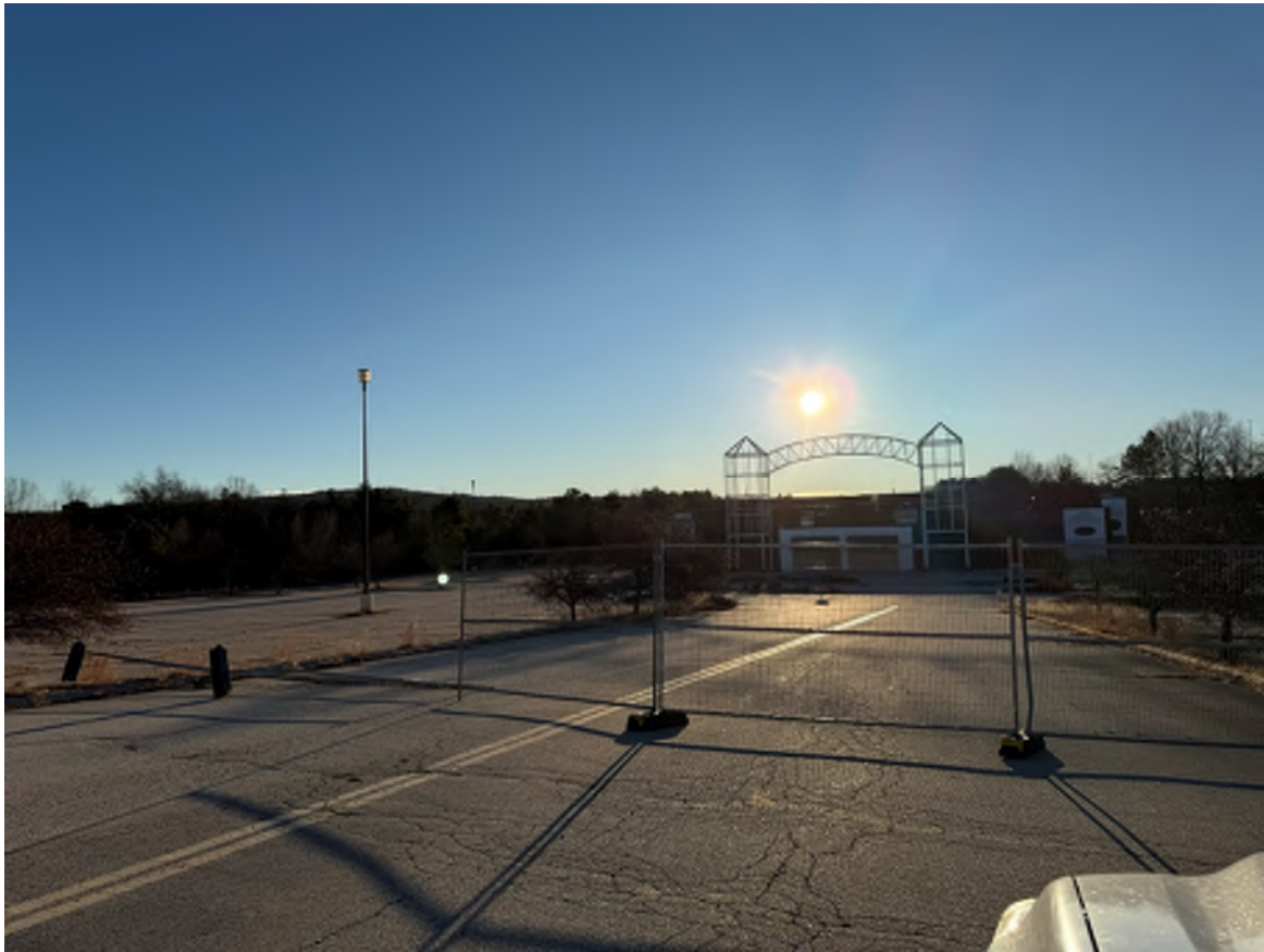
Photo 21: Looking East at the West side of Cinema (building to be razed).
