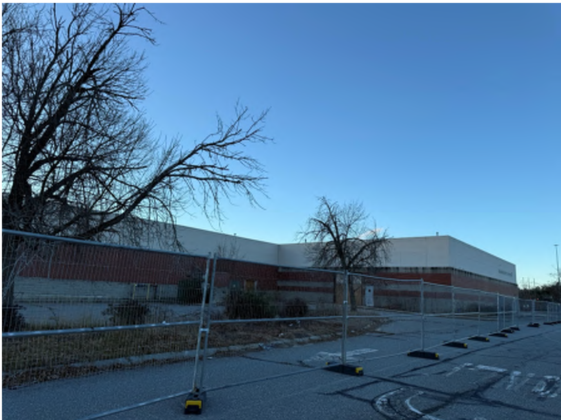
Photo 8: Looking Southeast at the West side of the mall (building to be razed).
