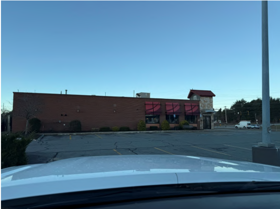
Photo 10: Looking South at the North side of Applebee's (building to remain).
