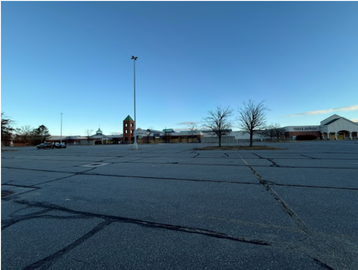
Photo 15: Looking North at the South side of the mall (building to be razed with the exception of the right side of the picture).
