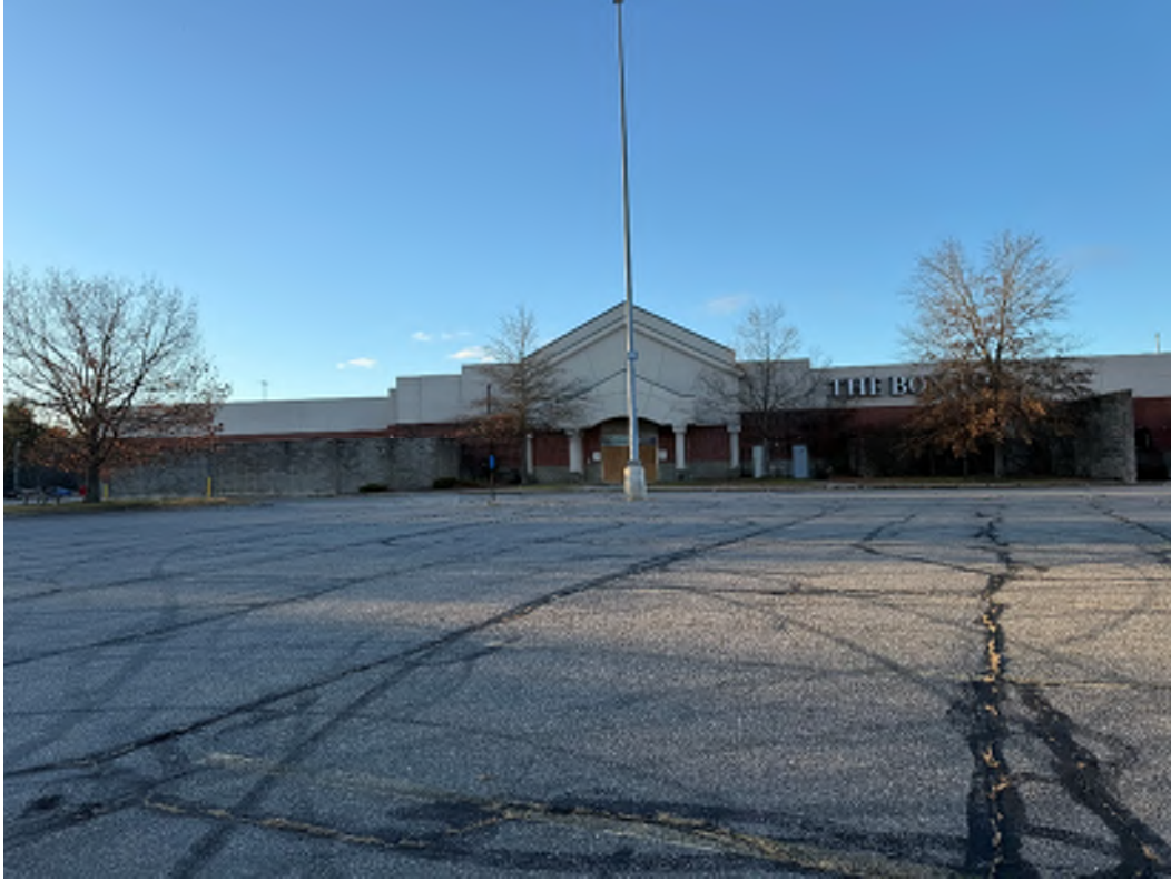
Photo 1: Looking Southeast at the North-East corner of the mall (building to remain).
