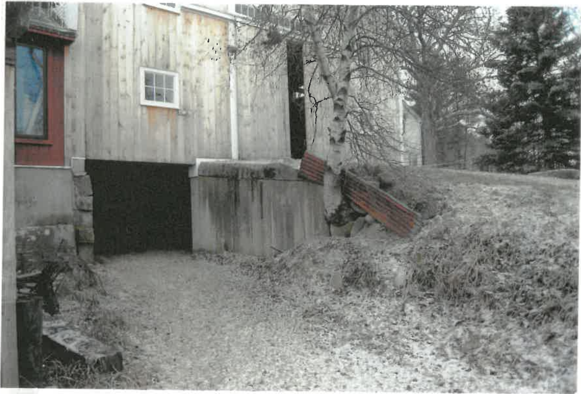
Entrance to barn cellar and ramp up to rear of barn
