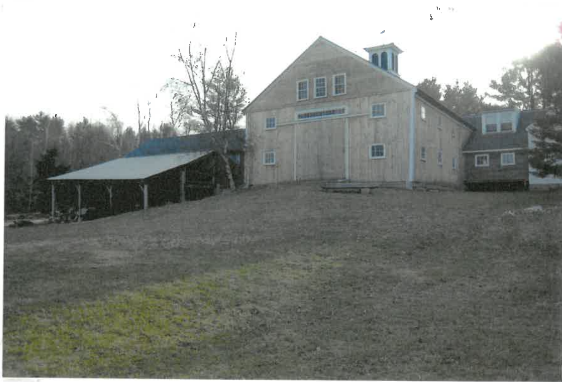
View from NE showing E side of barn
