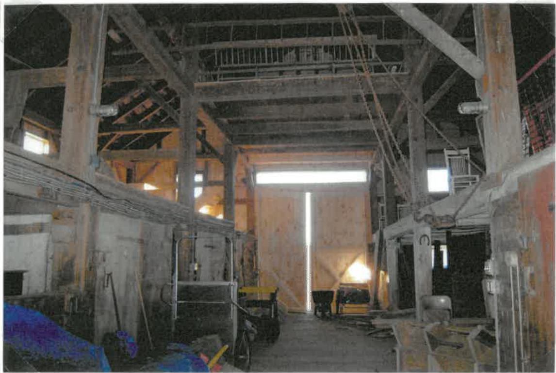
Main floor of barn looking towards the rear door
