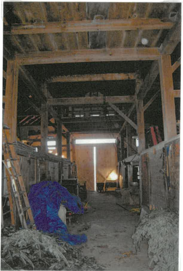
Main barn center aisle facing rear of barn
