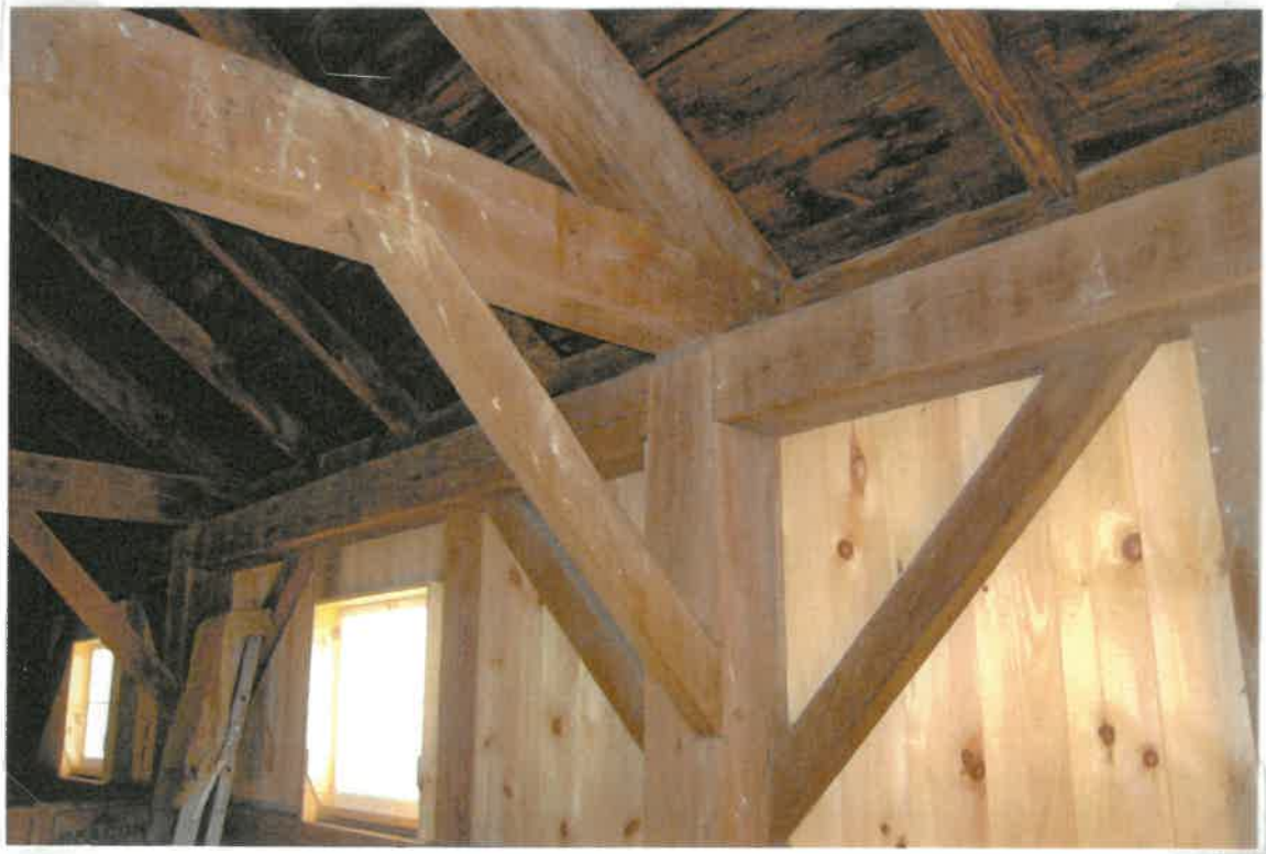
Post and beam
