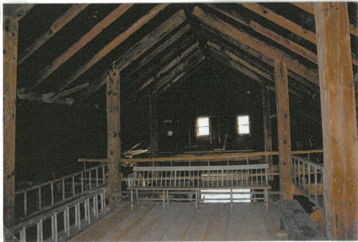
Third level of barn looking toward the front
