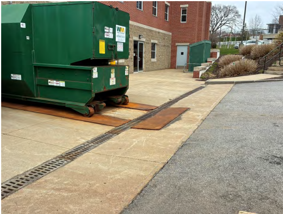
Photo #10 – View looking north at loading dock area.
