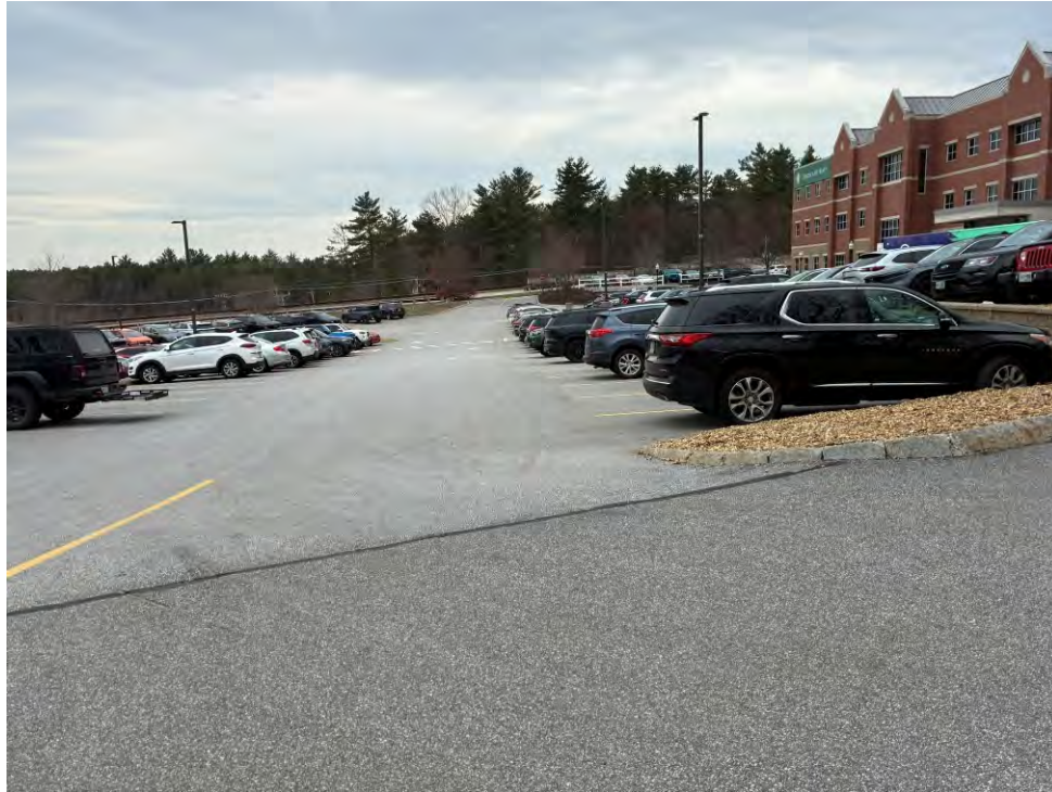
Photo #1 – View looking west at parking lot south of the existing medical center building
