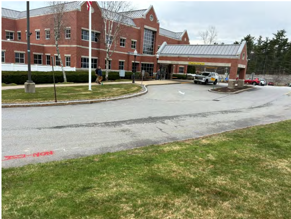
Photo #4 – View looking southwest at the front entrance of the medical center
