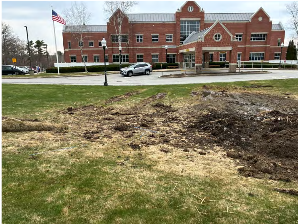
Photo #5 - View looking south at the front entrance of the medical center
