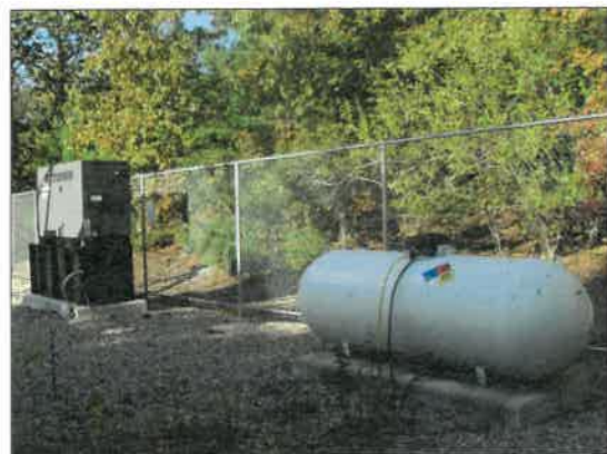
TYPICAL PROPANE GENERATOR NOT TO SCALE
