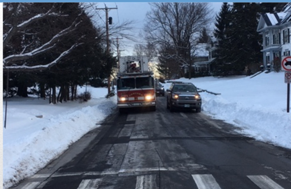
Pine Street (Warren to Pleasant) 30' +/- Wide; 2-Way Traffic 20 Parking Spaces (Both Sides) Potential Recommendation: Remove On-Street Parking on One Side
