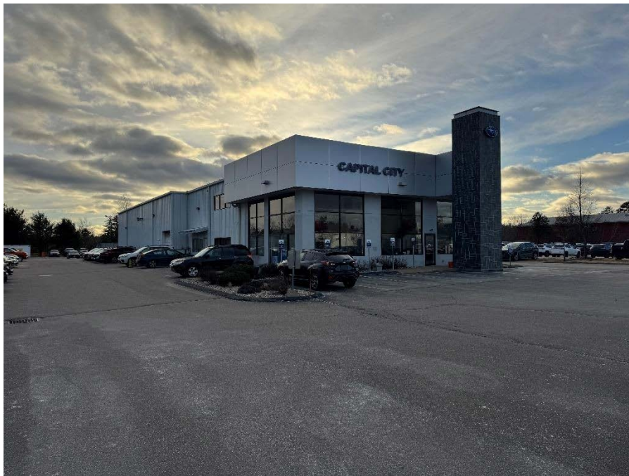
Picture 2: View southwest of the existing dealership roadside façade
