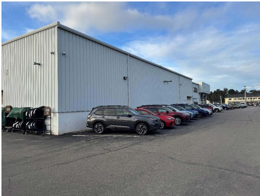
Picture 18: View of the eastern elevation of the exiting dealership
