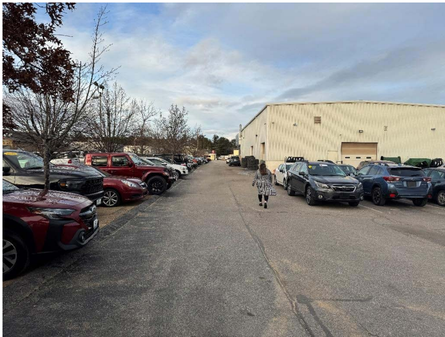
Picture 16: View from southwest corner of the parking area along the western elevation of the dealership
