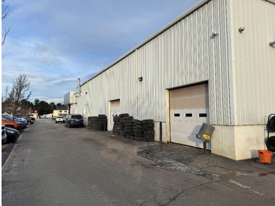
Picture 17: View of the western elevation of the exiting dealership
