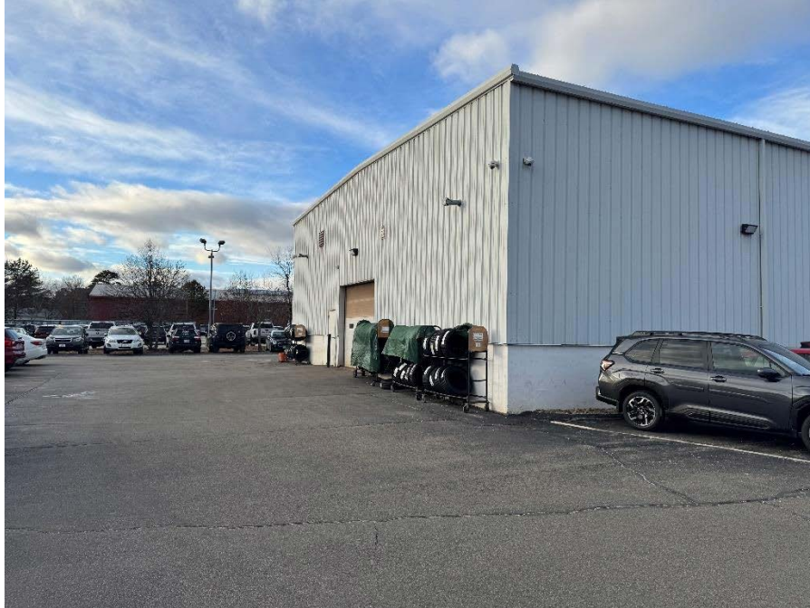
Picture 19: View of southern elevation of the existing dealership
