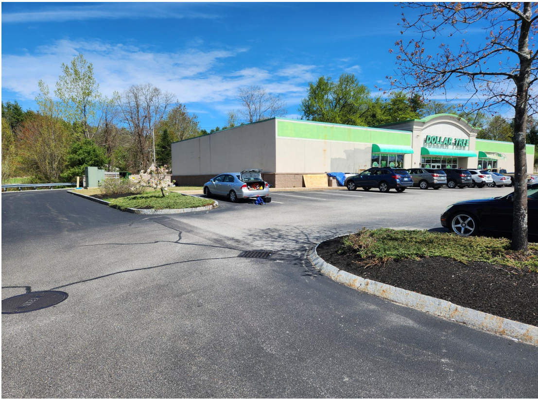
P1: EXISTING UNIT 2 AND FACE OF BUILDING FOR ADDITION
