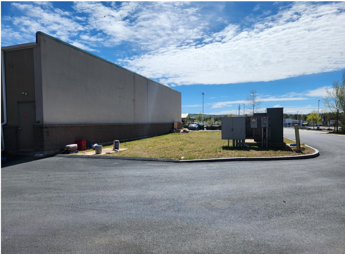
P4: FACING SOUTH ALONG FACE OF BUILDING FOR ADDITON.
