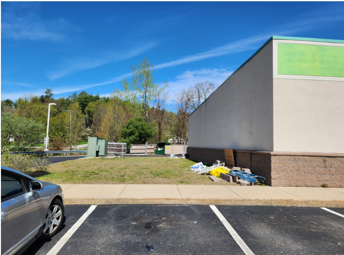
P2: FACING NORTH ALONG FACE OF BUILDING FOR ADDITON.
