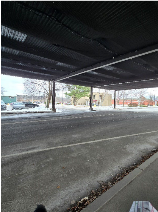
Vehicle access viewed from Storrs Street
