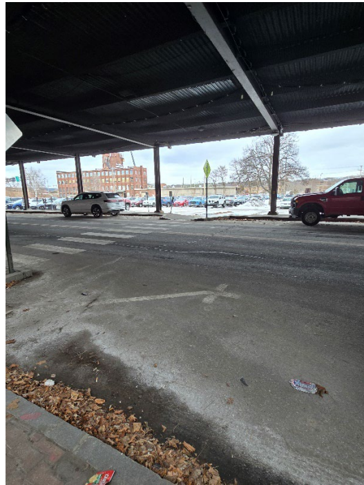
Primary pedestrian access from Storrs Street
