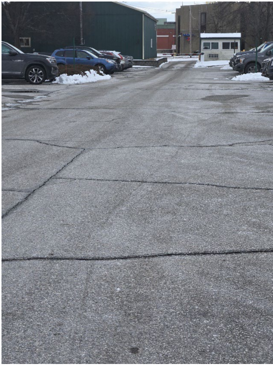
View south to vehicular access
