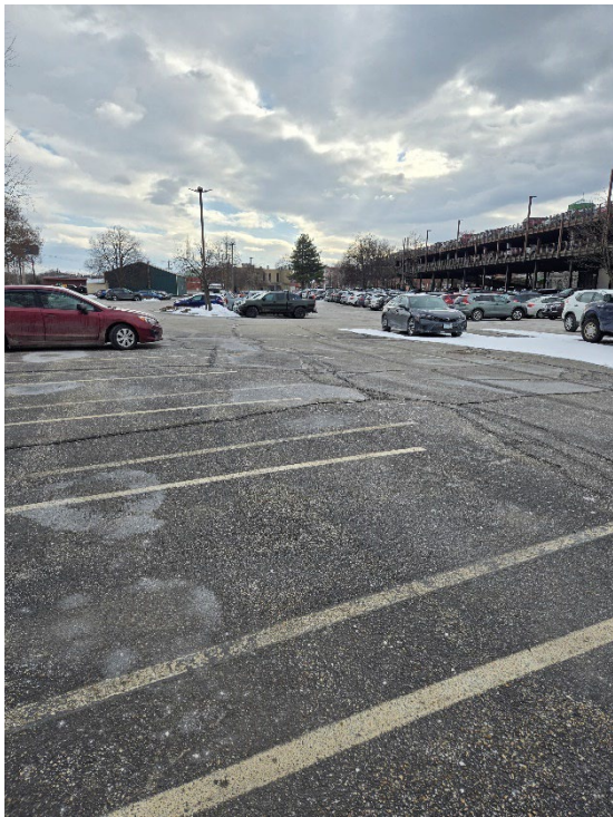
North lot viewing south
