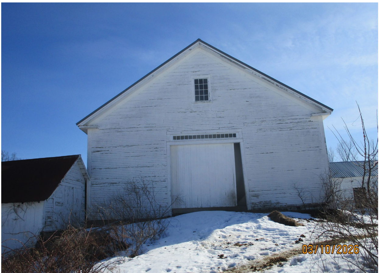
Rear (north) Side
