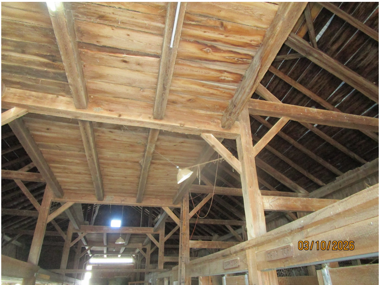
Flying Scaffold *Note Knee braces
