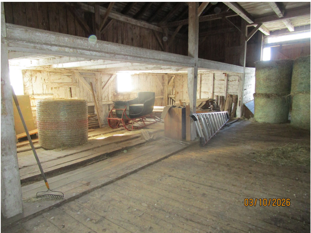
Northwest Side Loft
