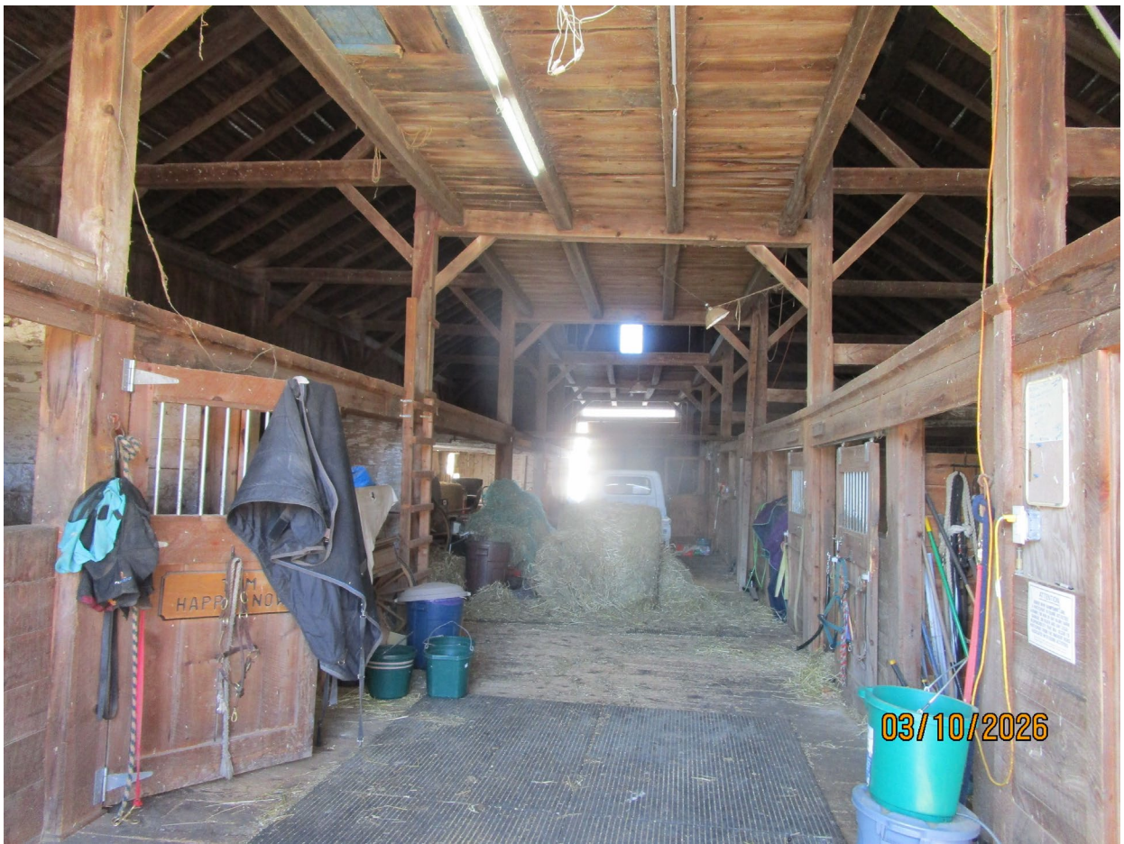
Interior View from Front
