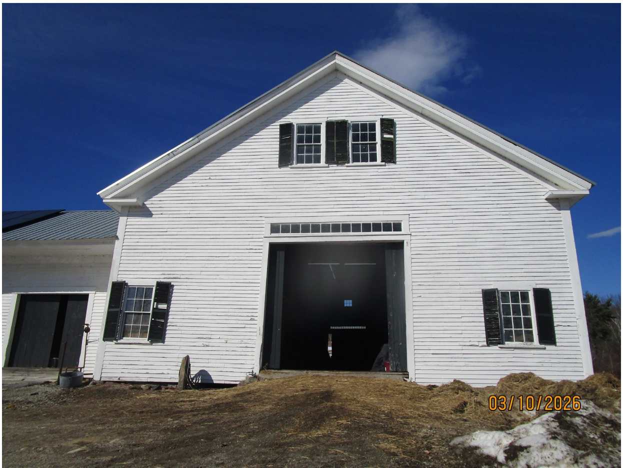
Front (South) Side
