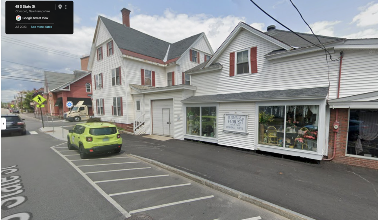
Existing Overhead Door to interior loading area (view looking north)
