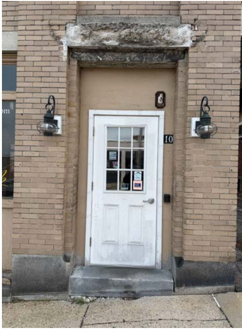
Old door location (Pleasant St Ext side of building)
