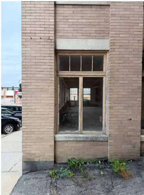
New door location (In the alley)
