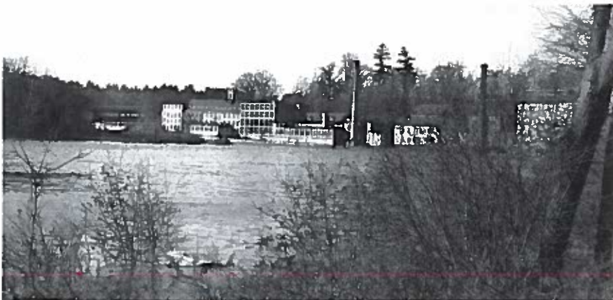
Harris Mill by the river in lower Boscawen – Harris house is top of the hill – left of center Steam Chimney.
