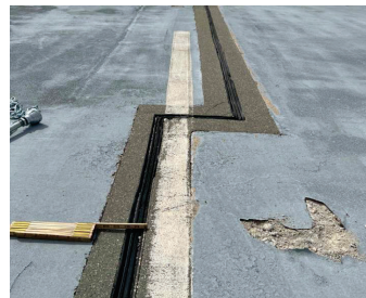
Expansion joint at roof level
