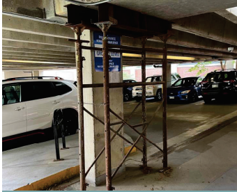
Shoring at one column (all levels)
