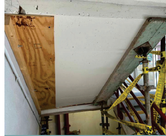
Shoring and plywood shields in stairs
