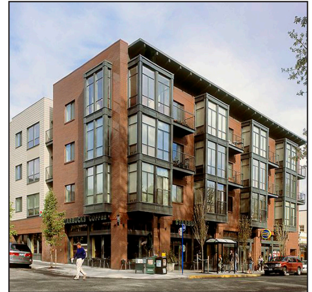
Balconies are recessed on a newer brick building with metal and glass architectural features that blend well with the balconies and are not within the right of way.
