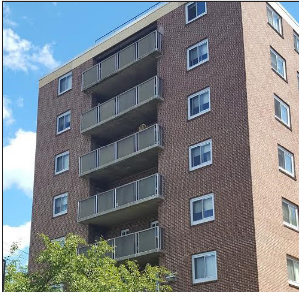
These inset balconies were part of the building's original design. Furthermore, they do not overhang the public right-of-way.
