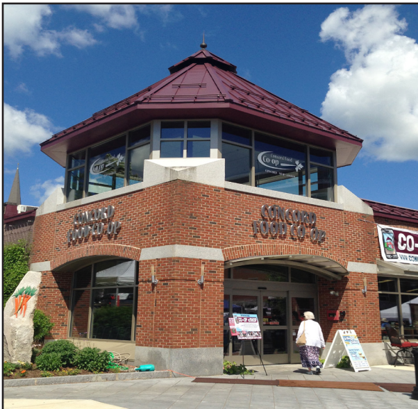
Different or modern architectural styles can be compatible with the community character and create a sense of vitality.
