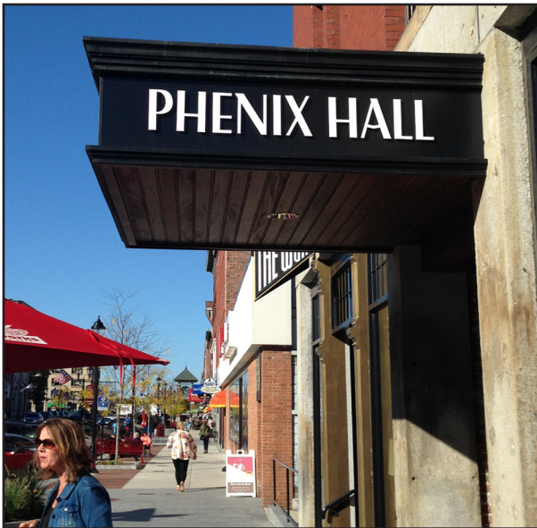
Canopies can help identify the building entrance and break up lengthy building facades.
