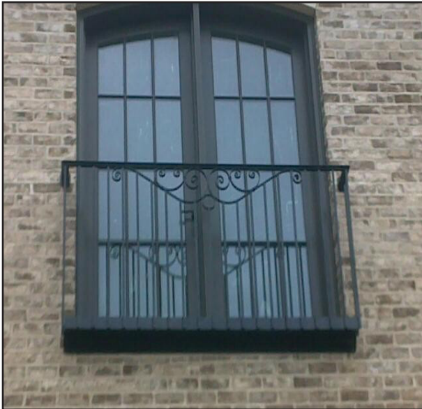
Elegantly designed Juliet balconies can provide private amenities without encroaching into the right of way.
