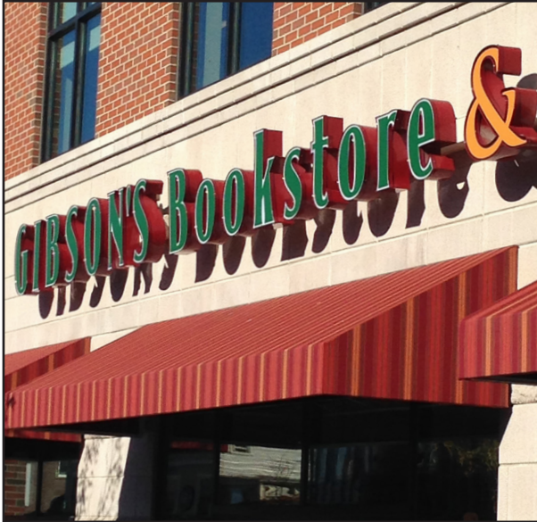
Awnings have long been a popular means to provide color and shade. This contemporary example complements the building and storefront.
