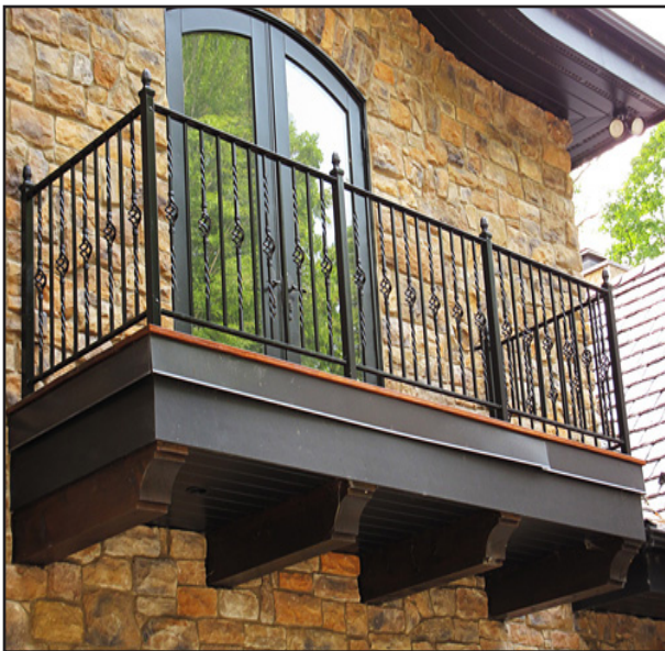
This retrofit balcony presents an attractive treatment of the underside.
