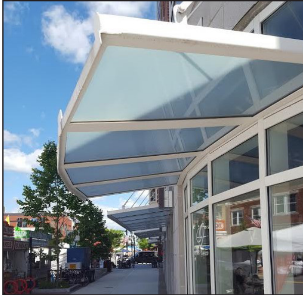
The clear glass of this canopy, placed on a modern building, complements the architecture and creates an interesting statement along the sidewalk.
