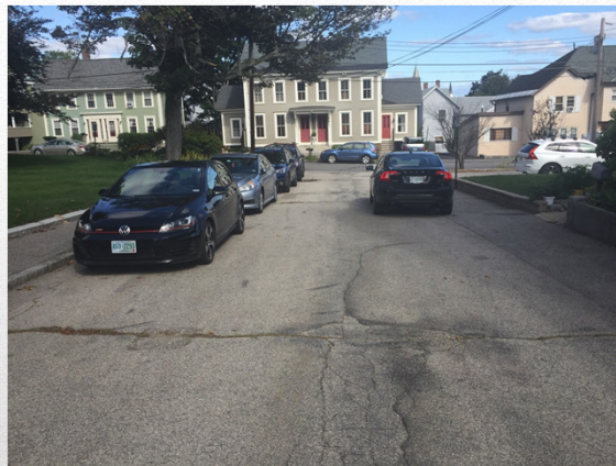
Garden Street (Huntington to Rumford) 21-23' +/- Wide; 2-Way Traffic 4 Parking Spaces (North Side Only) Parking Committee Recommendation: No Change 16
