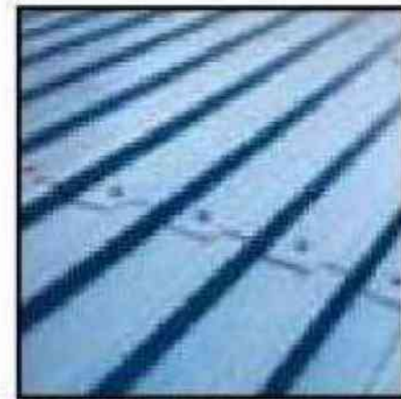
Standing Seam Metal Roof
