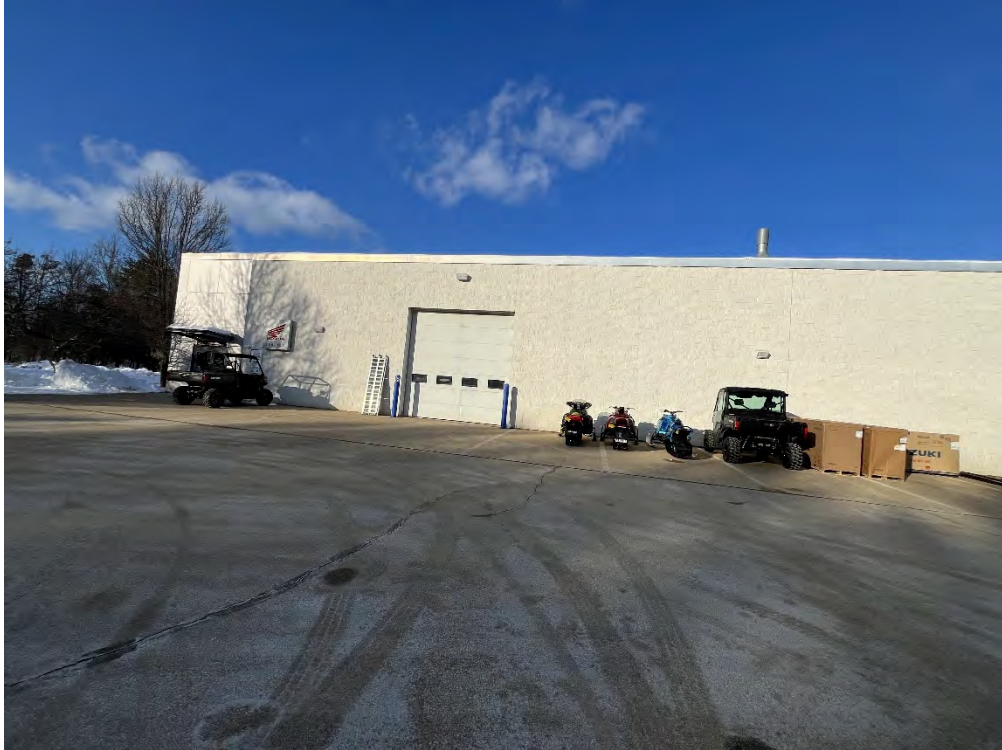
Figure 5: Southern side of Service Building (01/29/2026).
