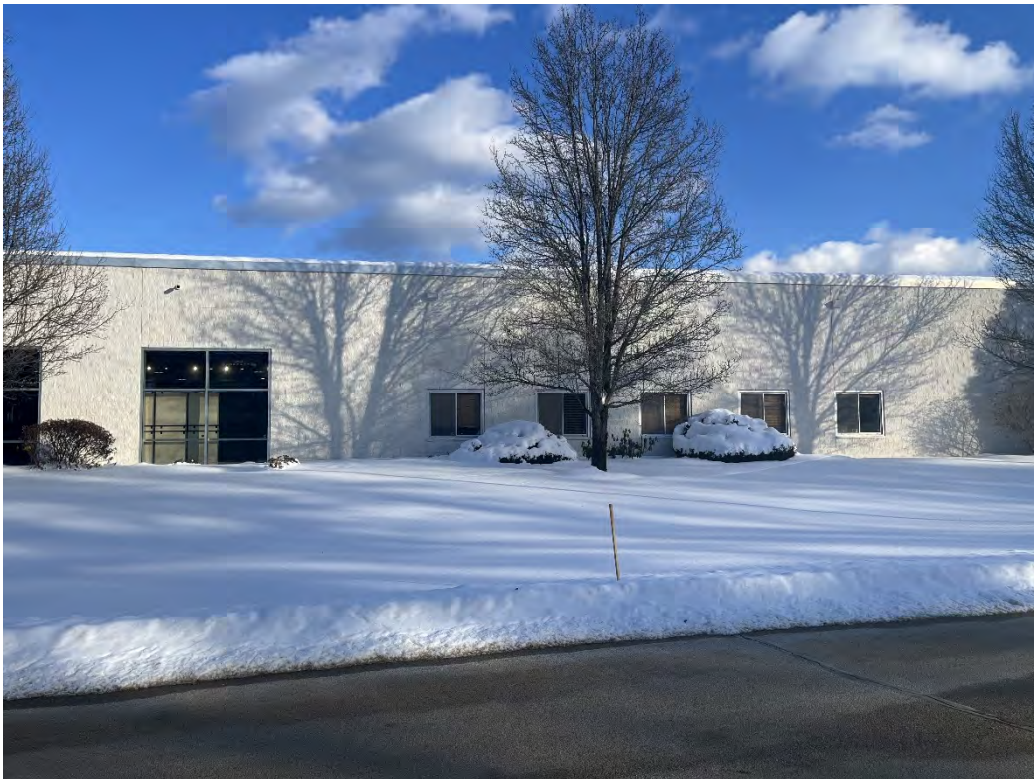
Figure 6: Western side of front building to be redeveloped (01/29/2026).
