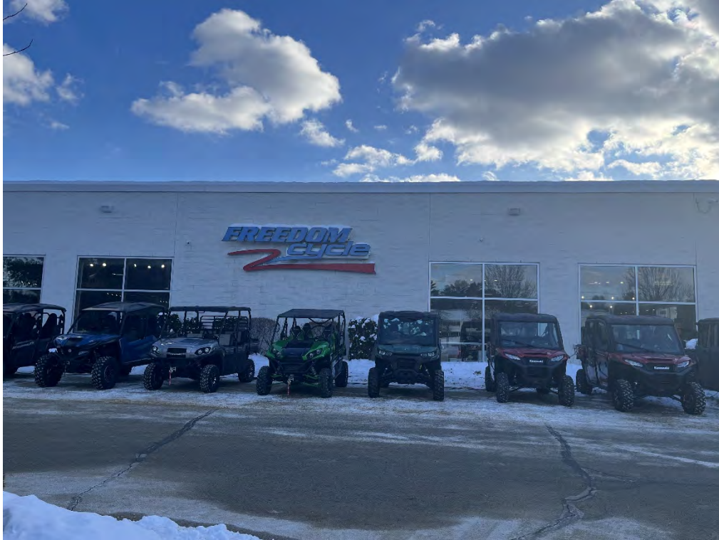
Figure 3: Existing building front façade (01/29/2026).
