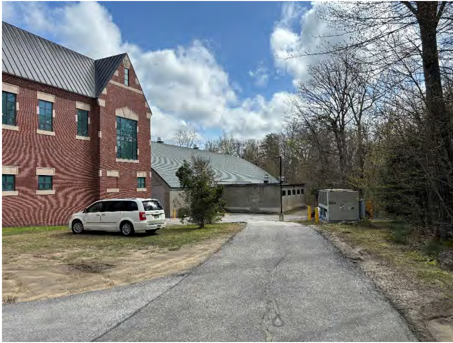
Photo #4- Back View of existing main site area to the northeast
