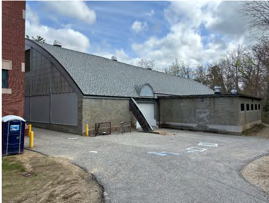
Photo #6- Back View of existing main site area to the northeast
