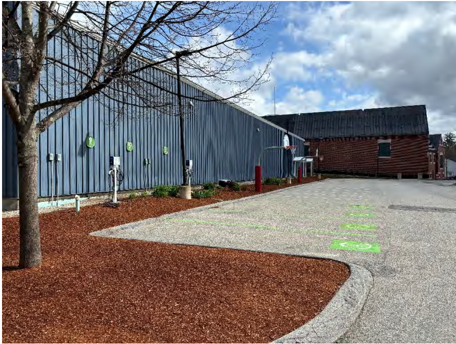
Photo #8- View of existing parking area to the northeast
