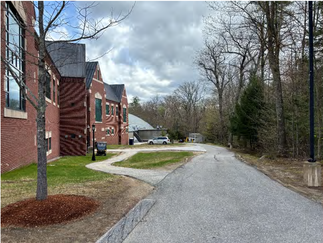
Photo #1- View of existing main site area
