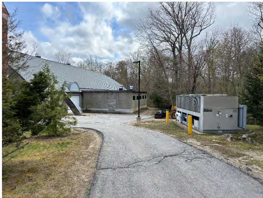
Photo #5- Back View of existing main site area to the northeast
