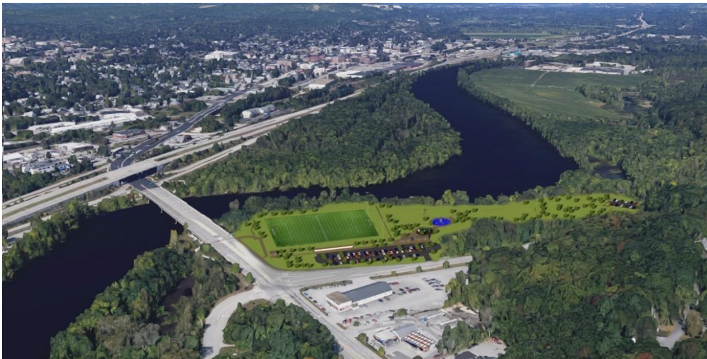
Aerial View of the new Terrill Park
