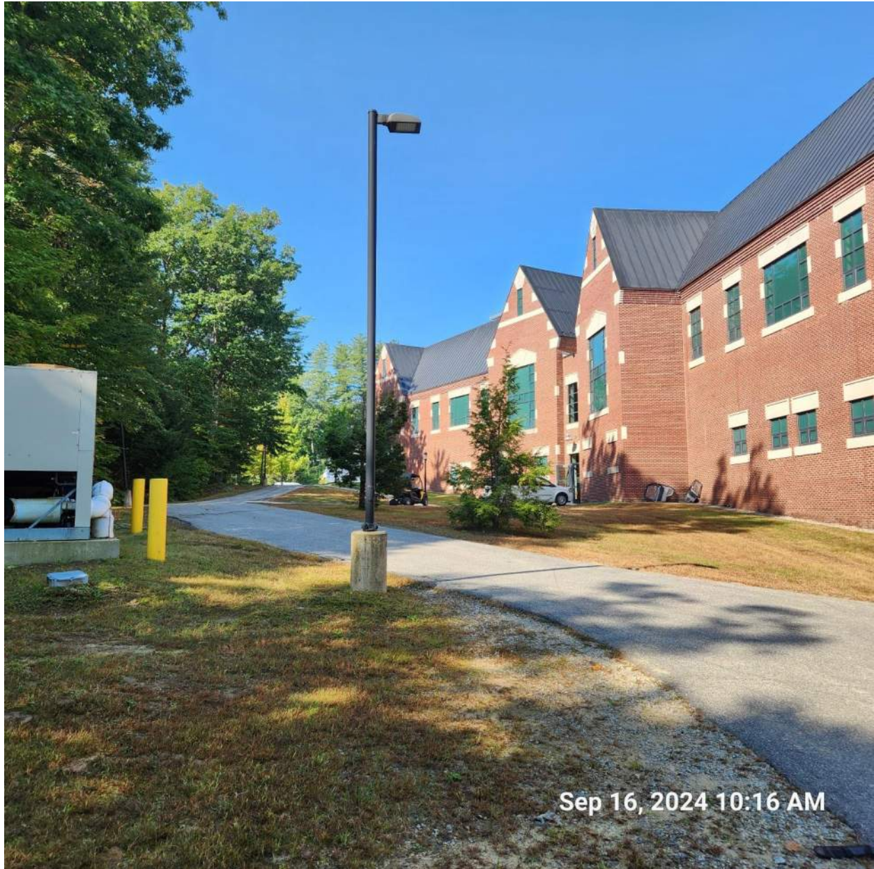
Photo #6: Looking west at proposed project location between the building and treeline.
