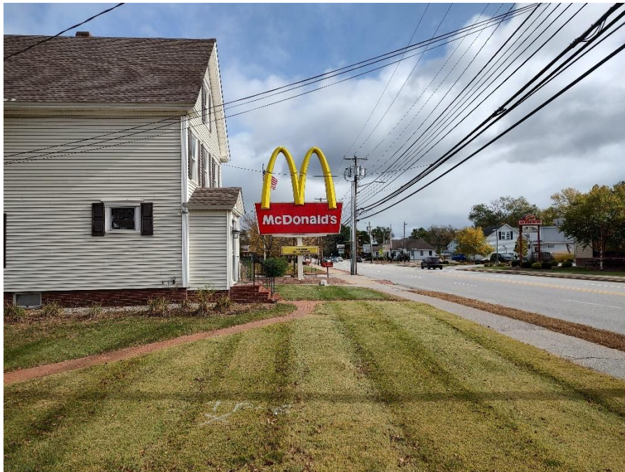
Photo #3- View of west side of site building
