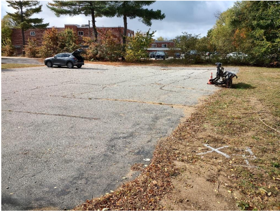
Photo #8- View of rear parking lot
