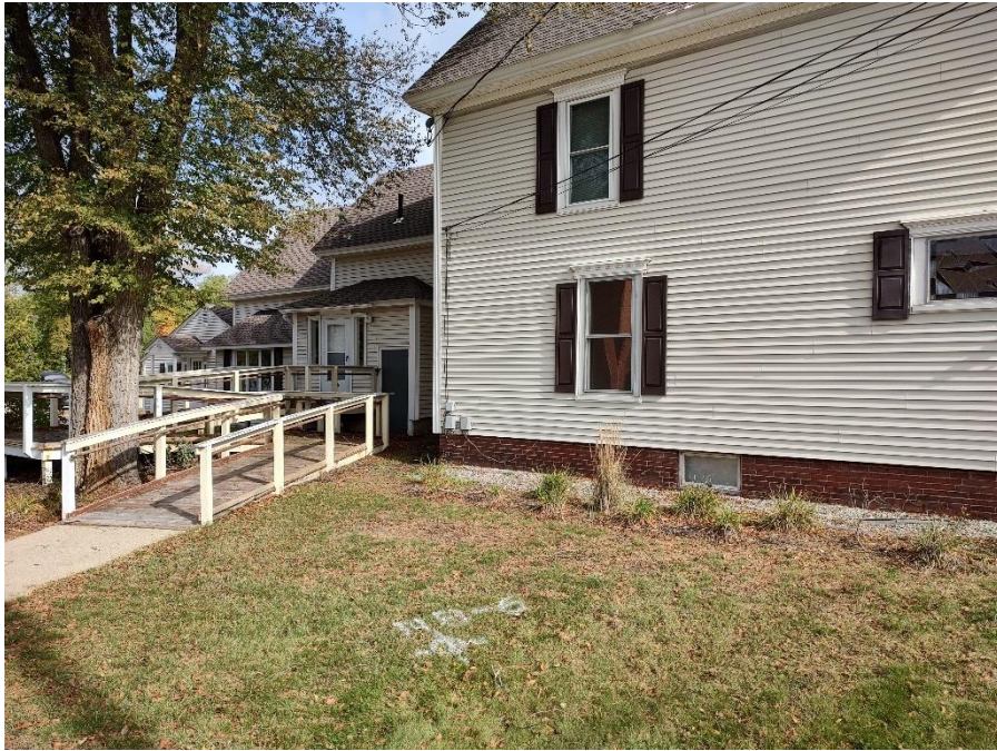
Photo #4- View of west side of site building
