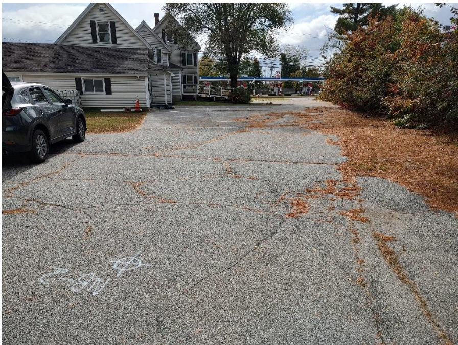
Photo #7- View of rear parking lot
