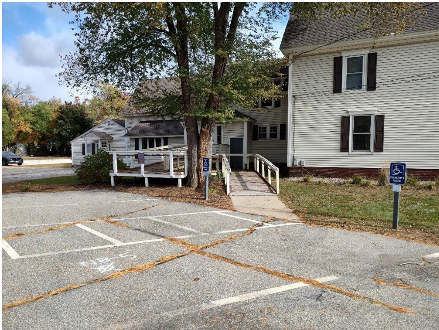
Photo #5- View of rear west side of site building
