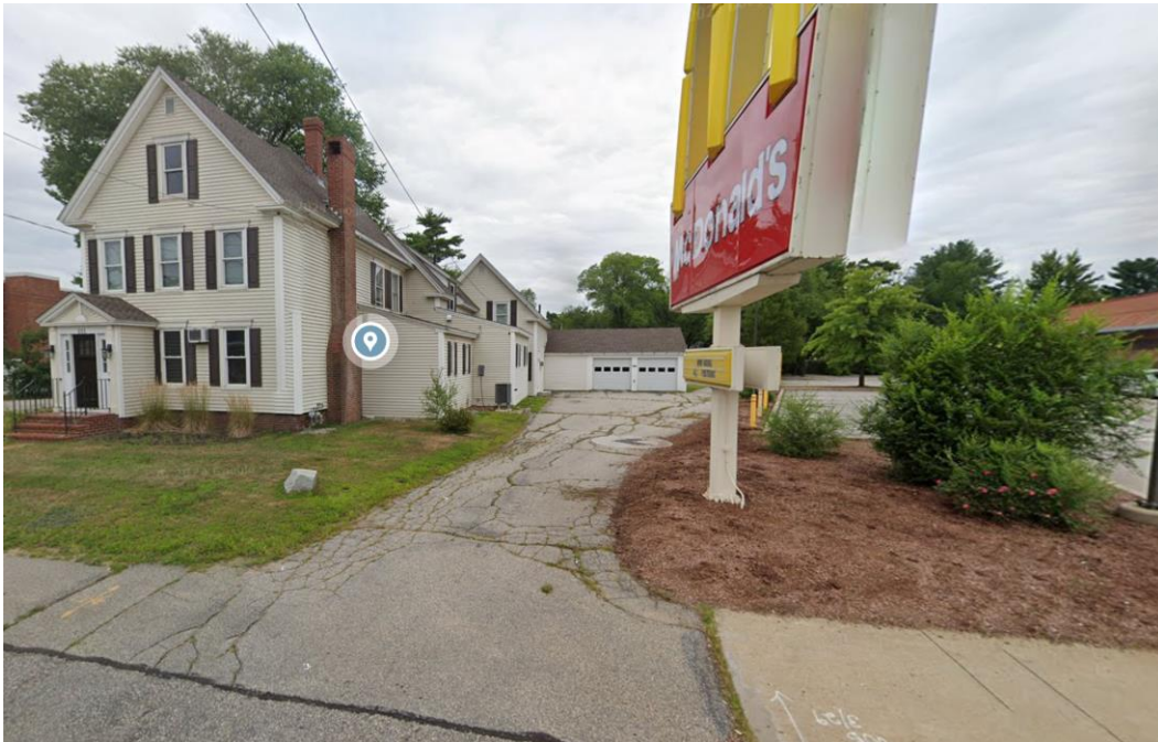
Photo #9-View of east side of site building
