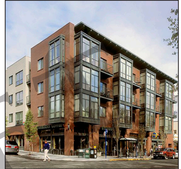
Balconies are recessed on a newer brick building with metal and glass architectural features that blend well with the balconies and are not within the right of way.
