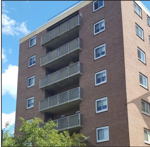
These inset balconies were part of the building's original design. Furthermore, they do not overhang the public right-of-way.
