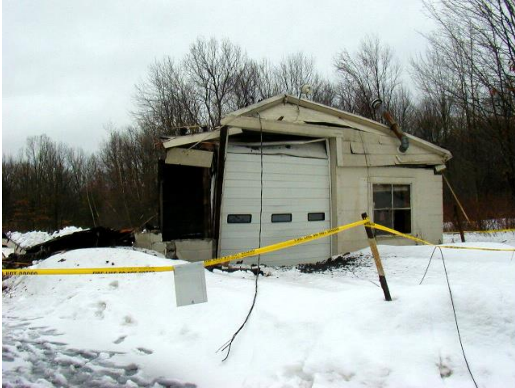
Building collapse due to snow loading on Elm Street, January 2008.
