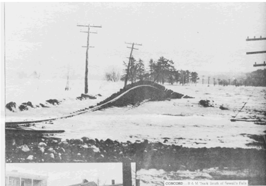
Railroad track damage at B&M Railroad Track south of Sewalls Falls, March 1936.
