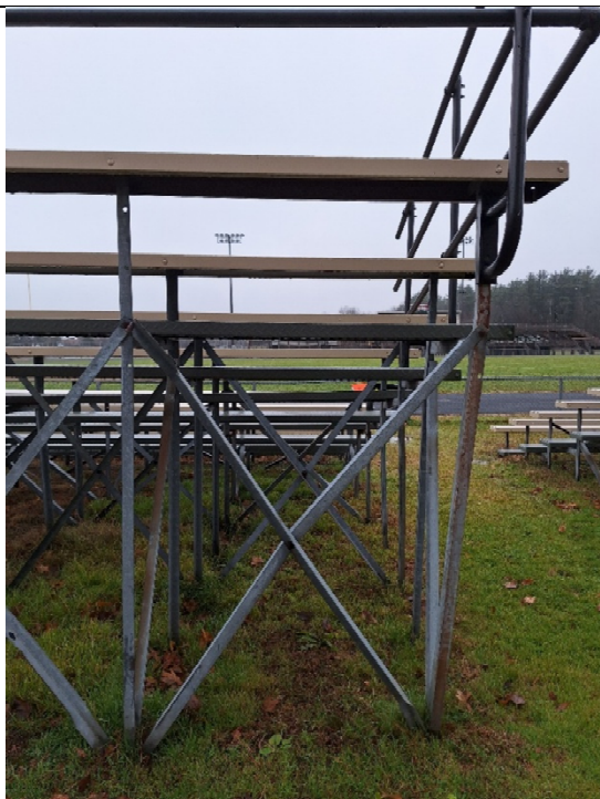
Photo 21 : Bent X Bracing, typical in many places.
