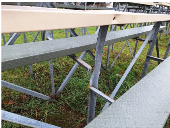
Photo 23 : Bent bracing and seating.
