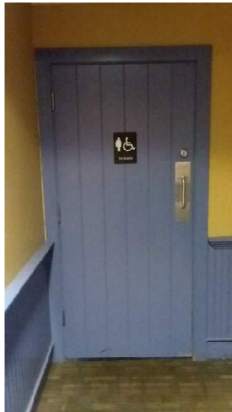
Accessible Restroom Signage Required on Wall Adjacent to Pull Side of Doors – Not Mounted on Doors
