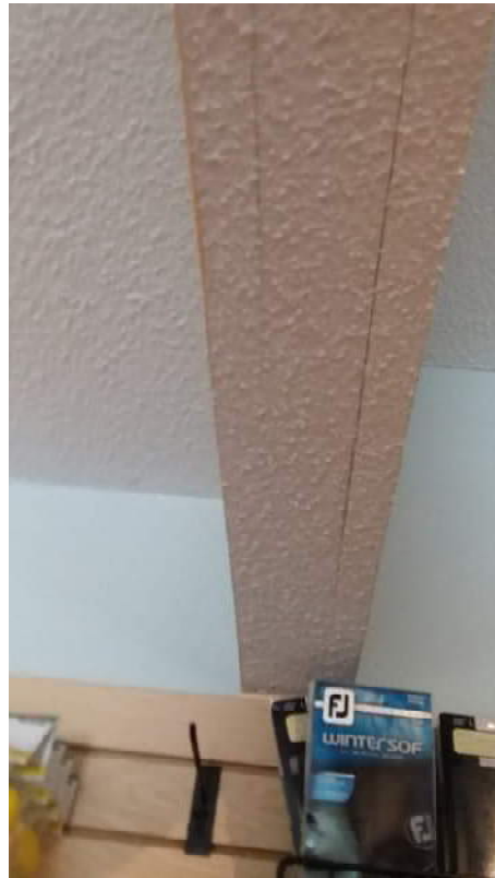
Beam Cladding Finish in Pro Shop
