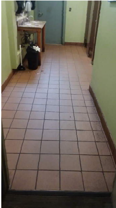
Tile Flooring in Restrooms
