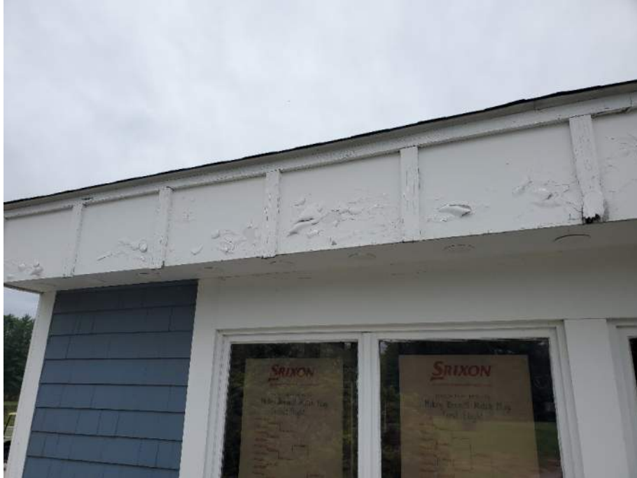
Roof Fascia on North Side
