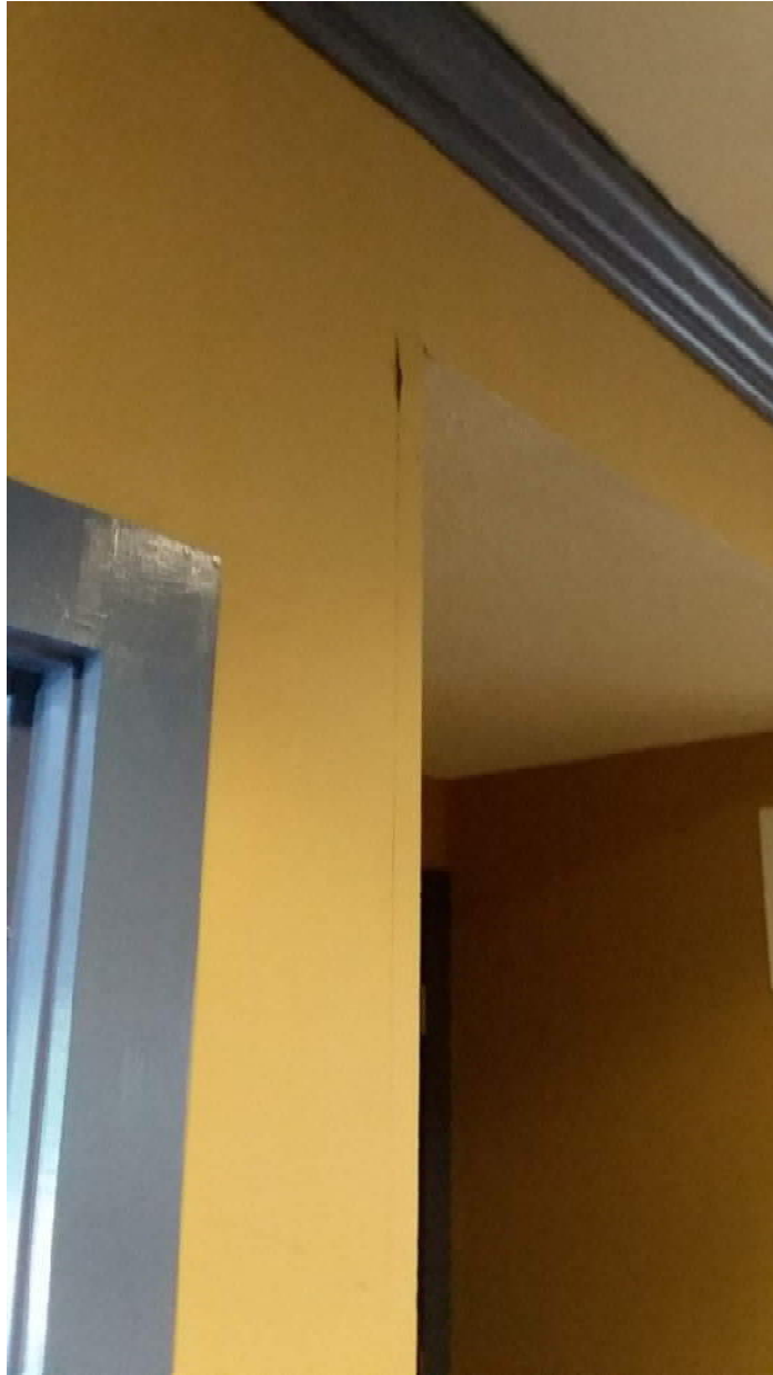
Wall Finish at Corner in Entry Hallway
