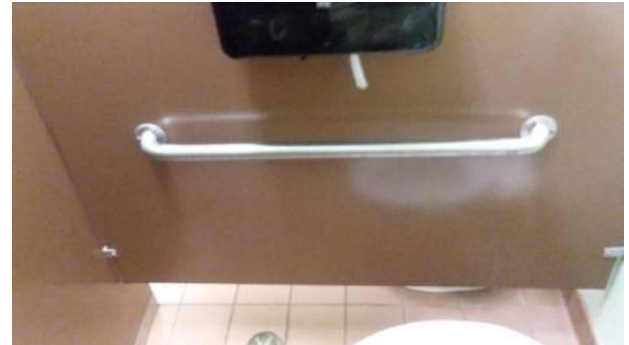
Missing Vertical Grab Bar
