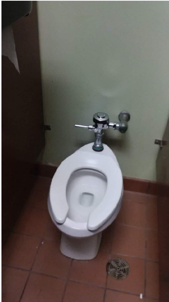
Compliant Smooth, Hard, Nonabsorbent Wall Surfaces Required within Two-Feet of Toilets & Urinals
