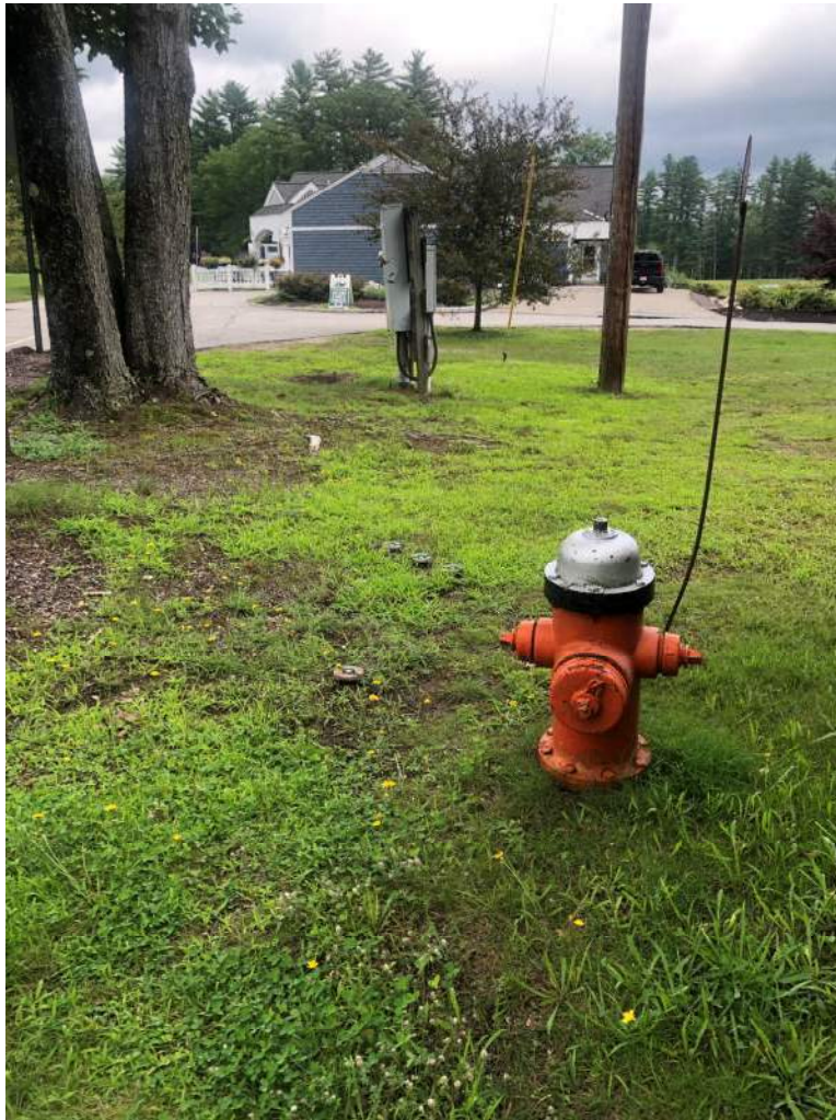
Water Hydrant and Electrical Service Located Southwest of Club House
