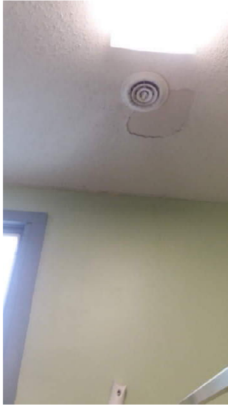
Ceiling Finish in Men's Restroom
