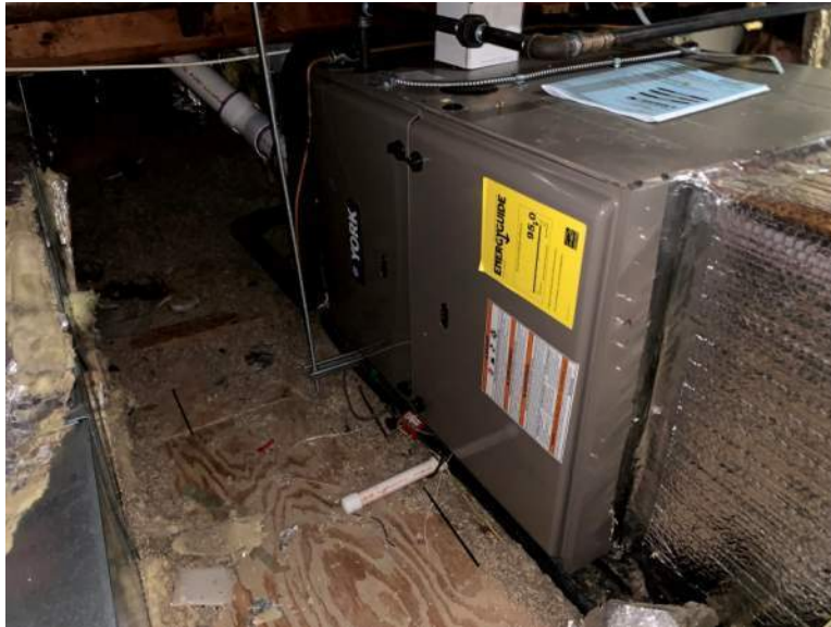
Function Room 5 ton air handling unit
