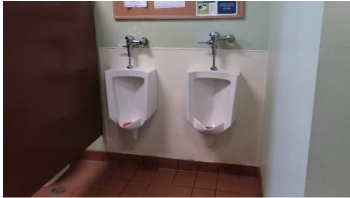
Compliant Smooth, Hard, Nonabsorbent Wall Surfaces Required within Two-Feet of Toilets & Urinals
