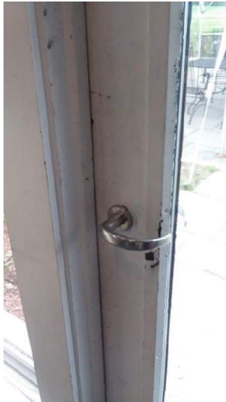
Interior of Exterior Door in Pro SHop
