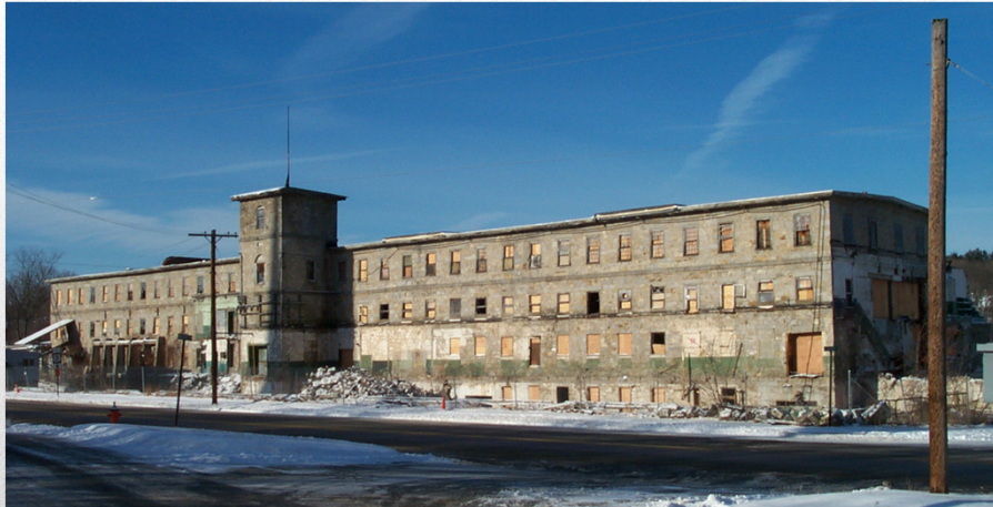
Penacook Mill Selective Demolition 2004/2005
