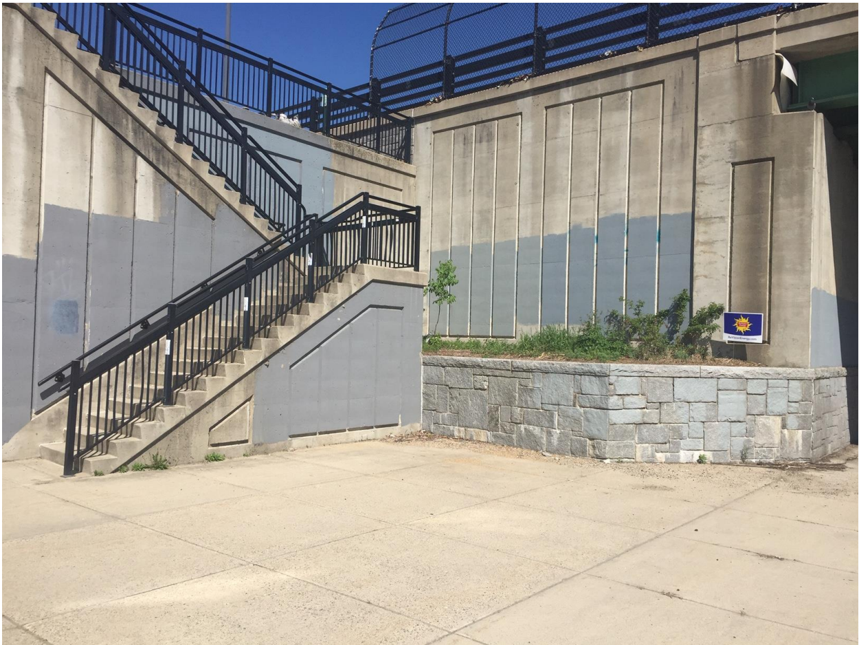
Photograph of Stairs and Associated Planter Box (Summer 2018)
