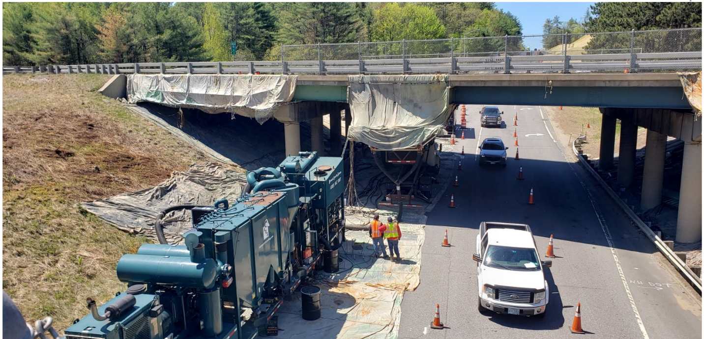
(Similar work at I-93 Exit 23 Meredith (2020))
